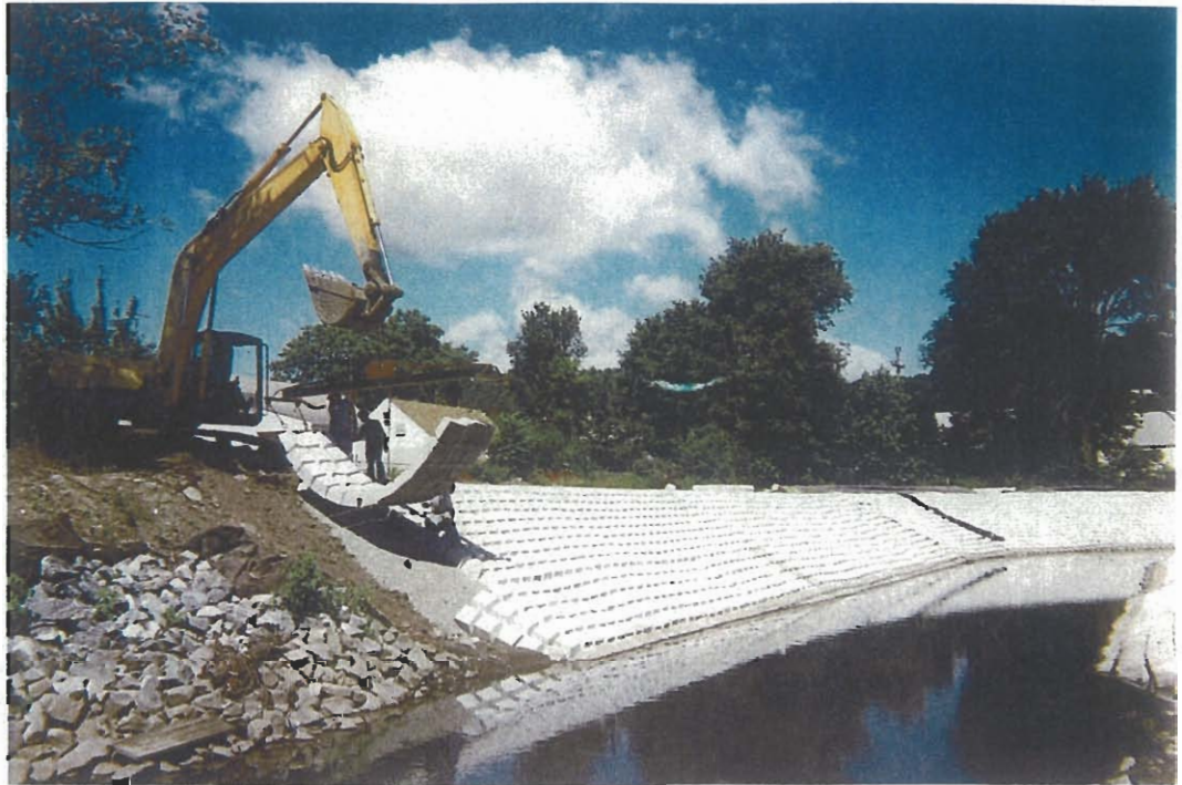
◄ Once the water level had lowered, an excavator installed mats from the bottom of the brook.
