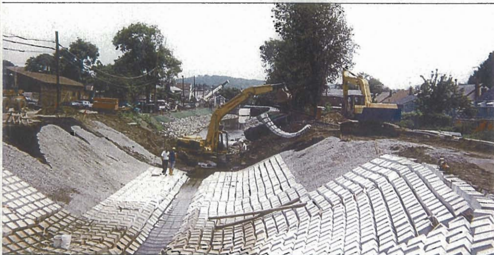
► The PC200 accommodated a spreader bar to place each cable mat.
