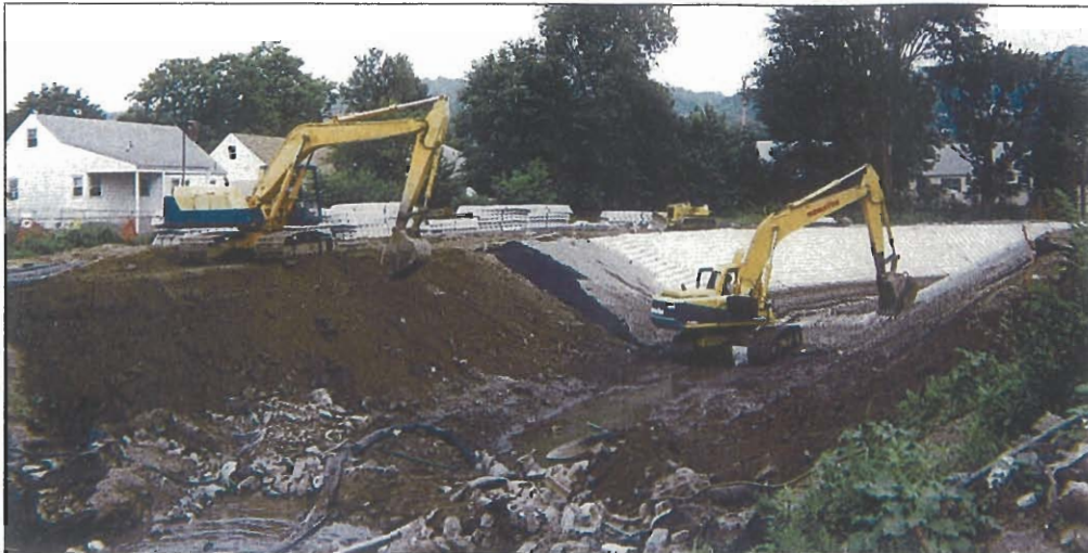
◀ From the top of the bank, a Komatsu PC200 excavator prepares the subgrade while another spreads three-quarter-inch clean stone.
