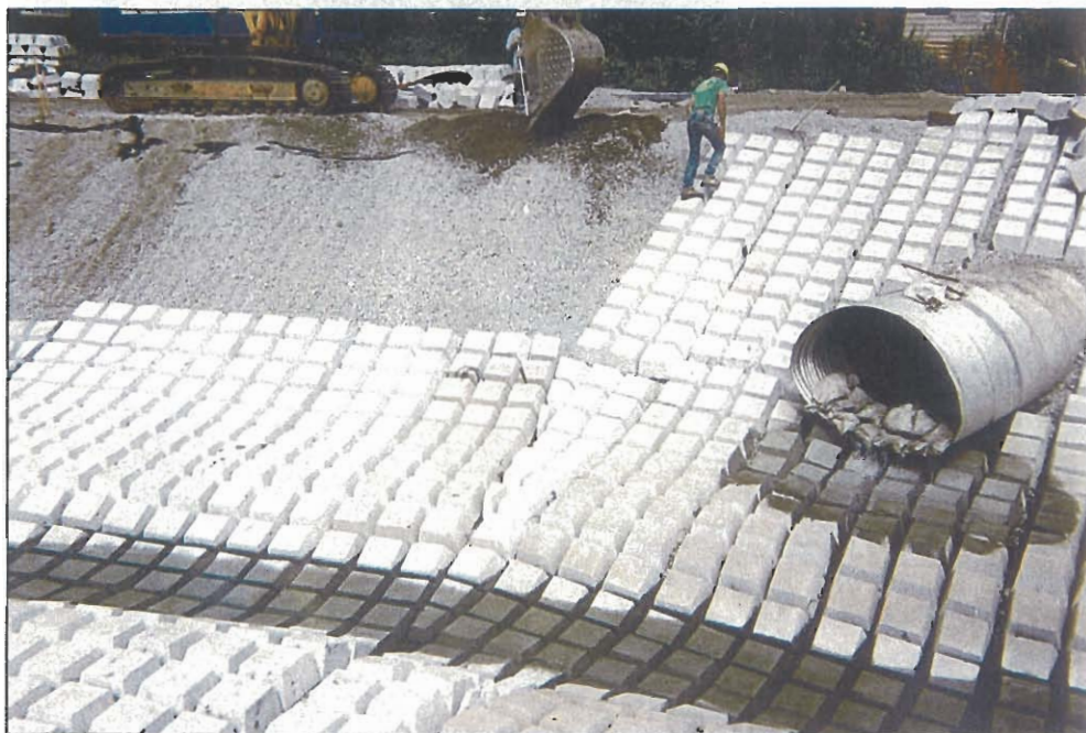
◀ From the top of the bank, a Komatsu PC200 excavator prepares the subgrade while another spreads three-quarter-inch clean stone.
